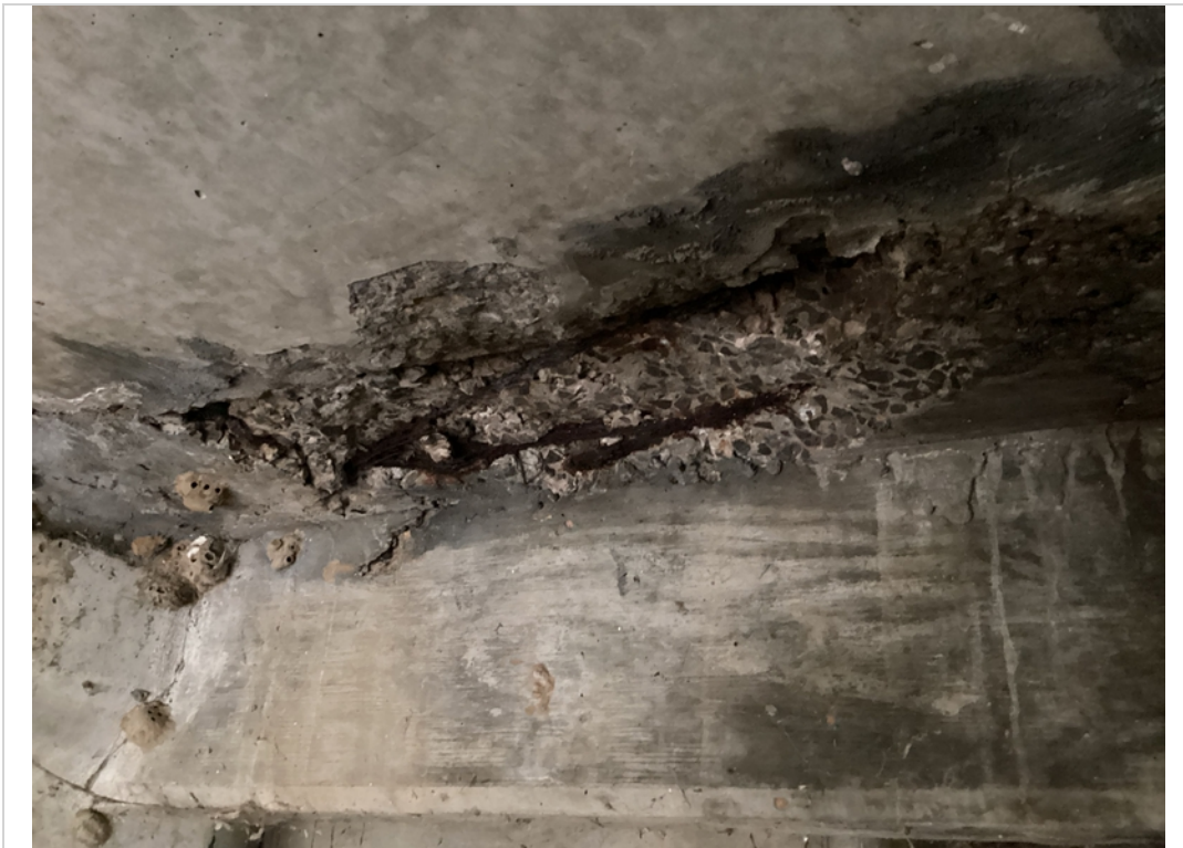
Bottom deck span 11A spalling to steel
