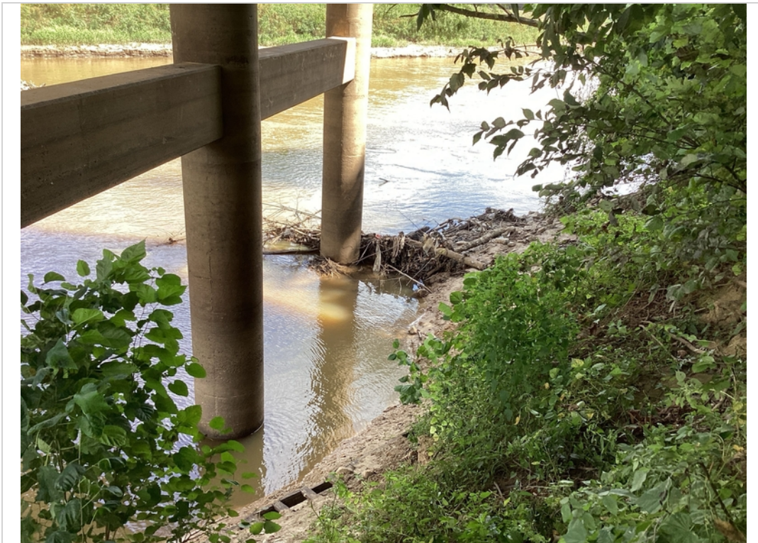
Bent 2 front side embankment washing
