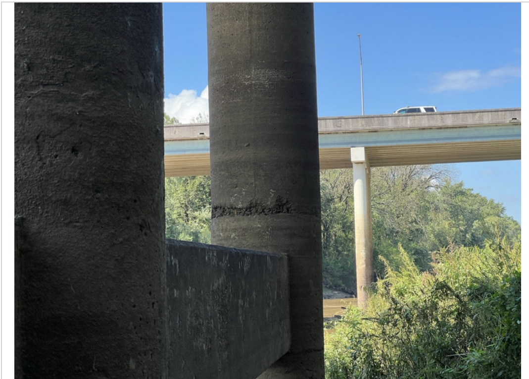
Bent 5 pile "A" abrasion
