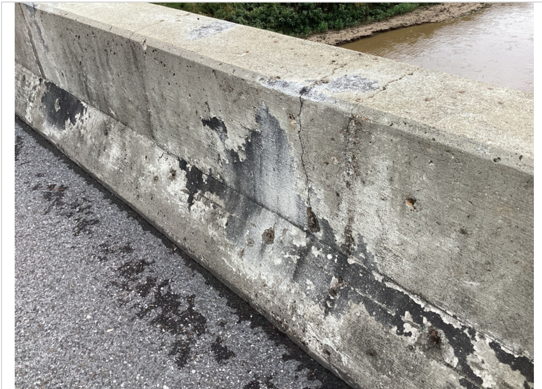
Span 3 , typical of parapet , cracks
