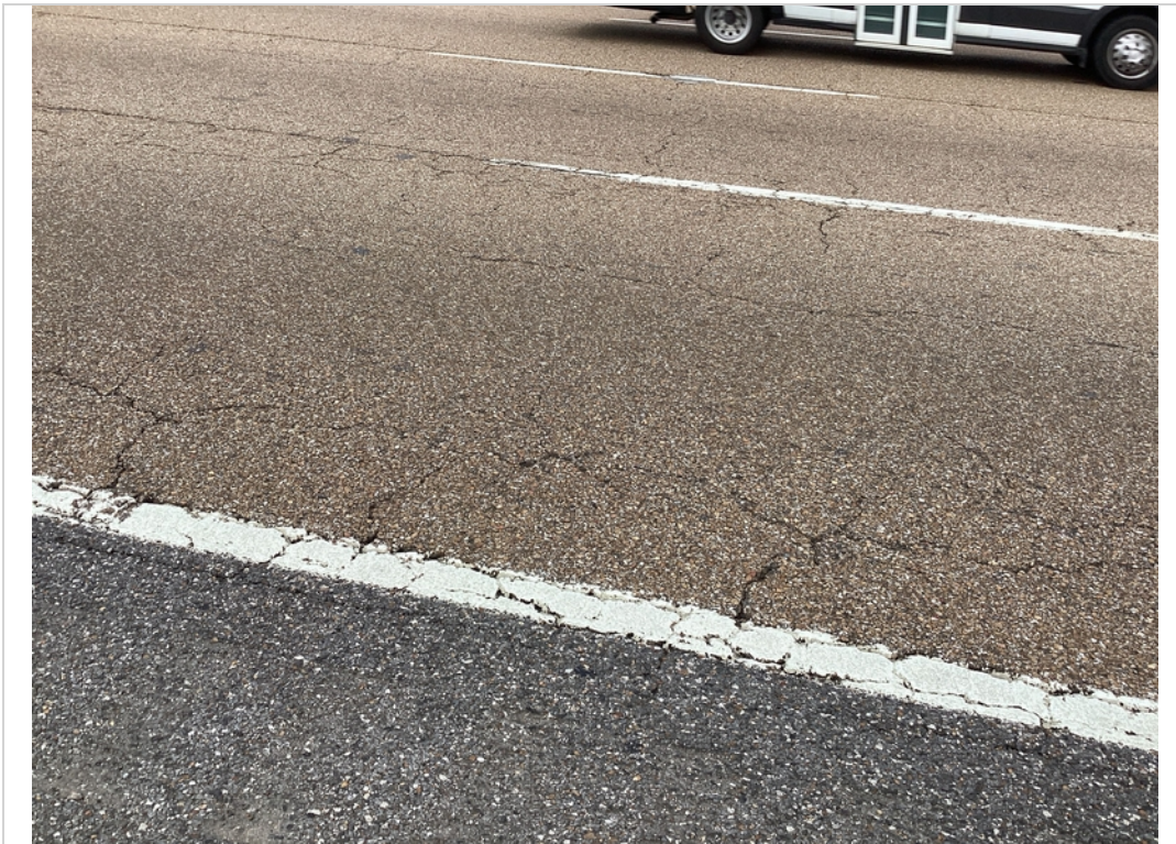
Span 3 cracks
