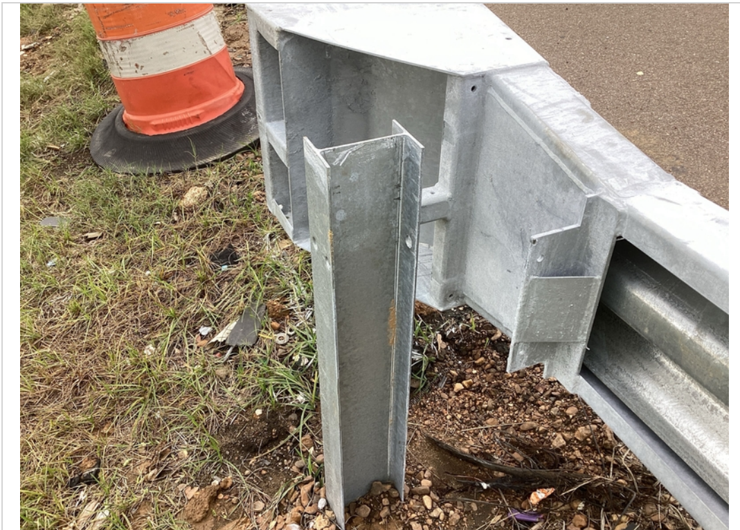
Approach 1 right terminal damage
